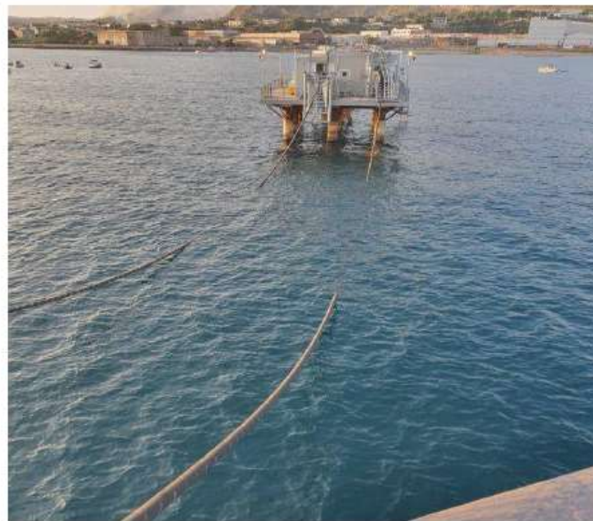
C2 HVDC Cable Load – LDV – Cable catenaries of both poles being well controlled between quayside and vessel.
