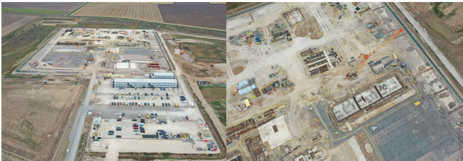
Overall view of platform facing north, attenuation pond, site accommodation,, contractors compound, AC haul road
