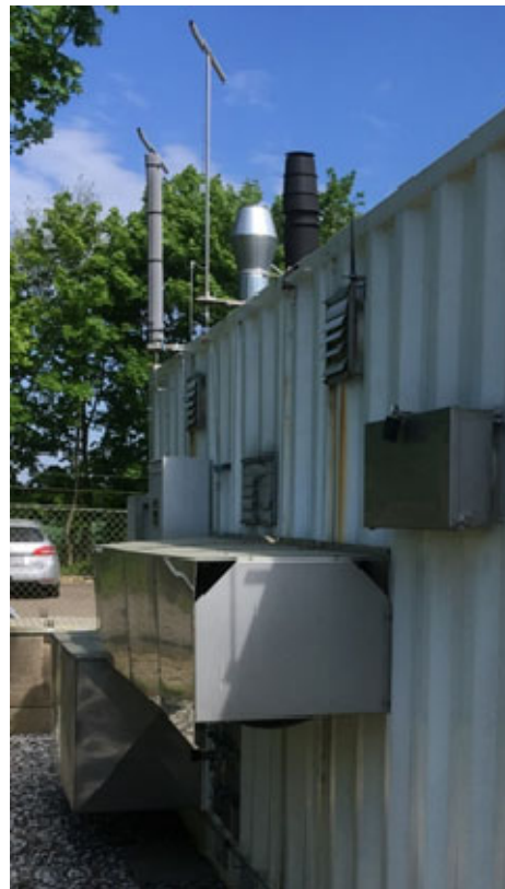
Figure 7. Hydrogen storage cylinder with protective cover.
