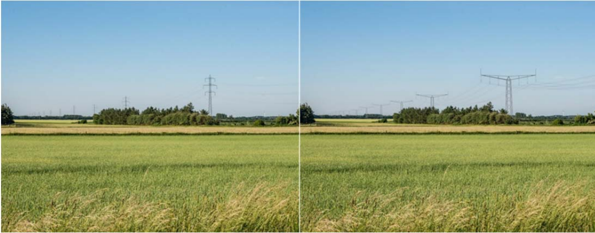
Figure 10 Left: Existing 150 kV OHL between Endrup and Idomlund. Right: Proposed 400/150 kV OHL.
