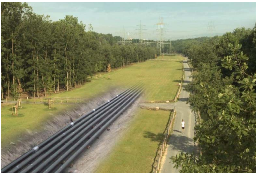
Figure 19: Two 400 kV GIL systems directly buried in Kelsterbach (photo: Siemens).
